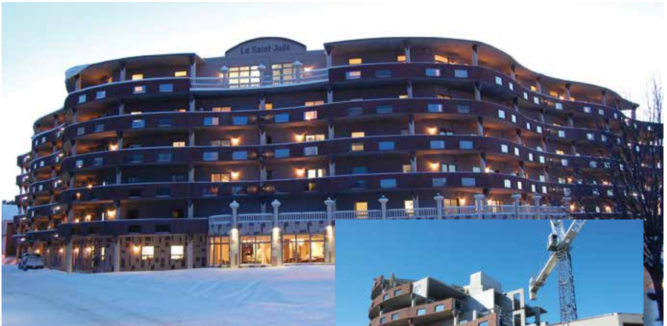
The Résidence Le Saint-Jude in Alma, Quebec, Canada used a total precast structural and envelope system to meet the project goals of this beautiful senior residence complex. Photo credit: Photos courtesy of Eric Painchaud, Architecte
