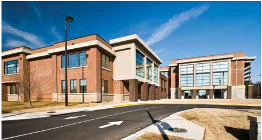
Tucker High School, in Tucker, Georgia, used a total precast system including columns, beams, double-tees, stairs, and insulated wall panels to complete this 340,000 sq. ft. project. Photo credit: Photo courtesy of George Spence, Metromont
