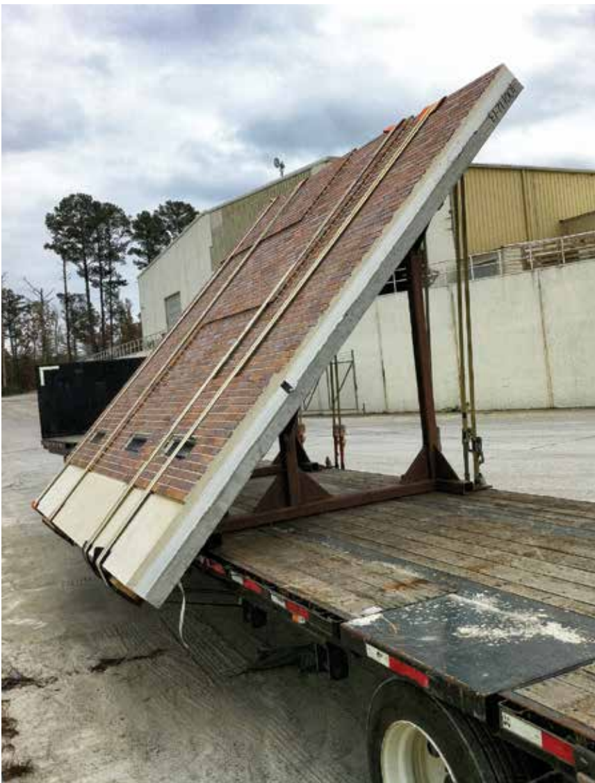
Continuous, edge-to-edge insulation is often used in precast concrete wall systems meeting ASHRAE requirements and helping to improve overall energy performance. Photo credit: Photo courtesy of Gate Precast Company
